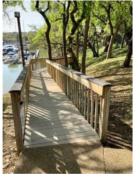
New marina deck completed in 2022
